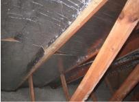
Attic showing reflective bubble wrap and cellulose insulation
