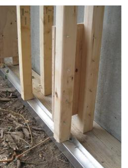
Ripped 2x4s down the middle & nailed together with plywood pieces the thickness of the desired wall cavity.
