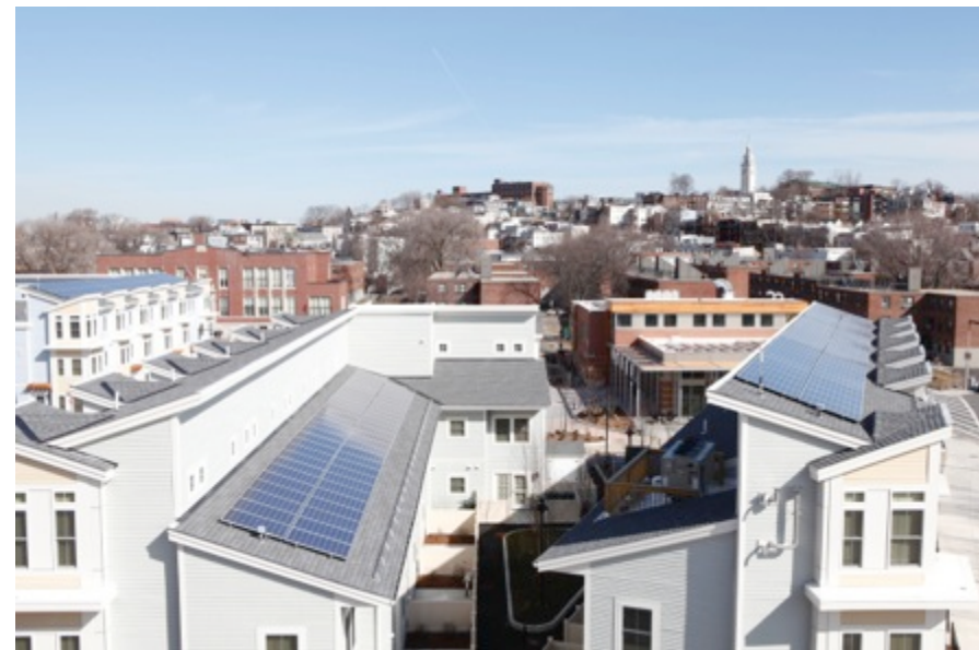
Old Colony affordable housing solar project in Boston
