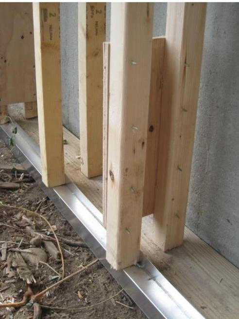
Ripped 2x4s down the middle & nailed together with plywood pieces the thickness of the desired wall cavity.
