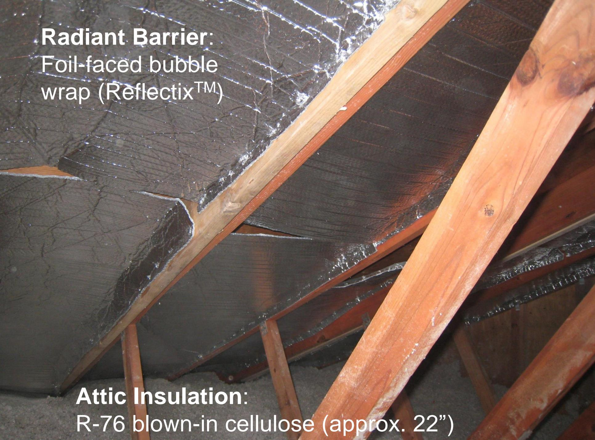
The image shows the interior of an attic. Several wooden rafters are visible, running diagonally across the frame. A dark, foil-faced material, identified as a radiant barrier, is installed over the rafters. Below the radiant barrier, there is a layer of insulation, identified as R-76 blown-in cellulose. The insulation appears as a thick, fibrous material filling the spaces between the rafters. The overall scene is dimly lit, with some light reflecting off the foil surface.
